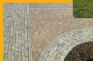
Variante in Betonstein
